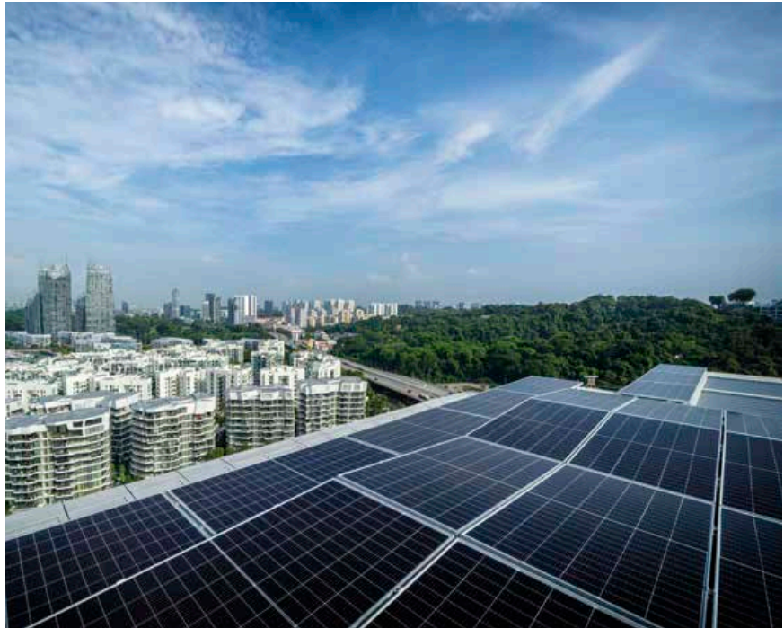
Installation of the photovoltaic panels at Keppel Bay Tower was completed in March 2021, generating an energy yield of about 100,000 kWh per annum.
